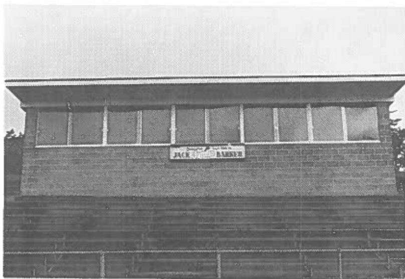
EDISON SOUTH'S NEW PRESS BOX
