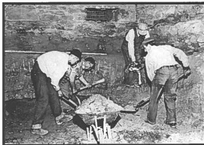
Excavation of Church Basement Jack Hamilton, Russell Giffin, Theodore Wise, and David Wise
