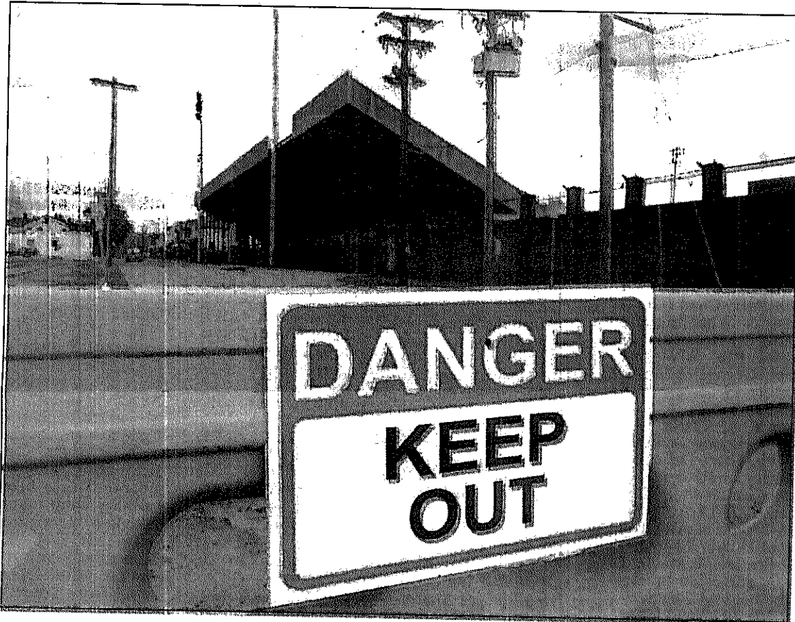
This section of South Penn Street remains closed because of structural problems at Wheeling Island Stadium.
