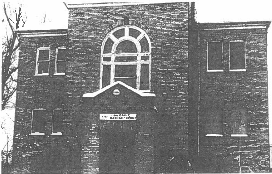
SITE OF THE FORMER DUN BAR SCHOOL
