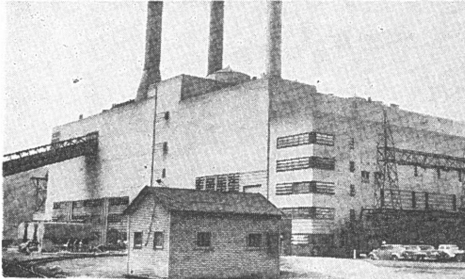
R. E. BURGER POWER PLANT of The Ohio Edison
